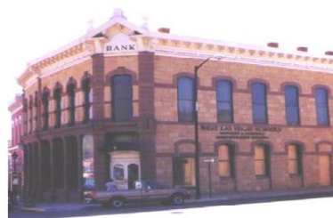
Example of a Bearing Wall Structure
